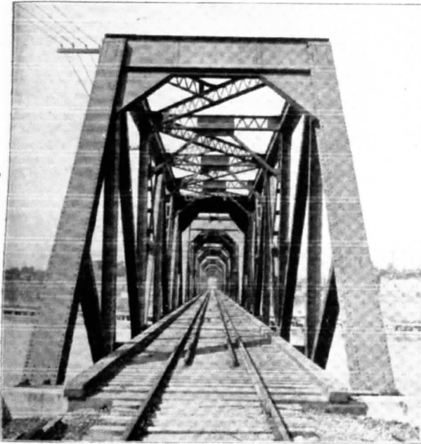
End View, Bay City Bridge.
